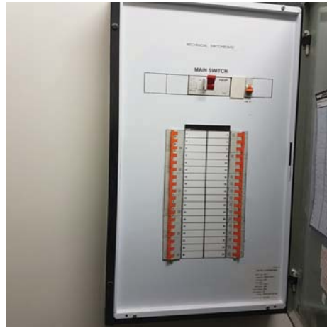
Residential switchboard upgrade and light upgrade Braeden H.
