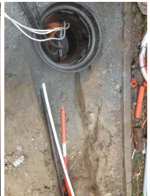
Installed underground supply and wired external structure Ellingworth
