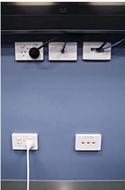
Light and power outlet upgrades Ben B.
