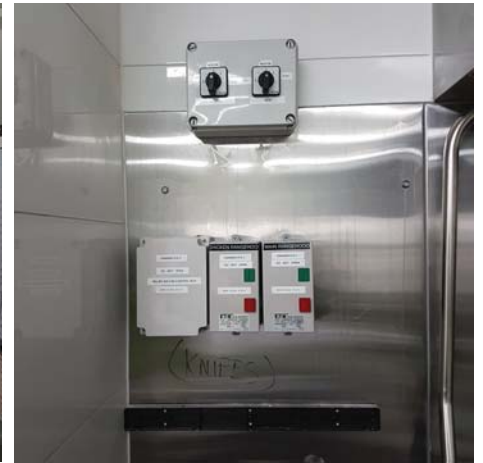
Mains and switchboard upgrade Helen S.
